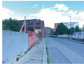
Via Cernaghola: The poor road conditions and the location of abandoned buildings make the area appear dangerous.
